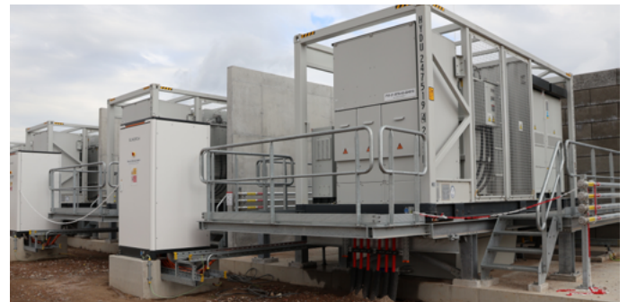
80 medium-voltage skids have been placed onsite
